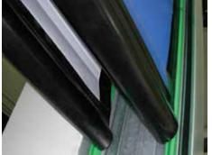
The dual-curtain design reduces frost build up — when closed, the two curtains create a dead air space which is treated with a small amount of heated air.
